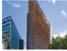
New Street Square, EC4 Innovative offices around a public square, with retail and restaurants.
